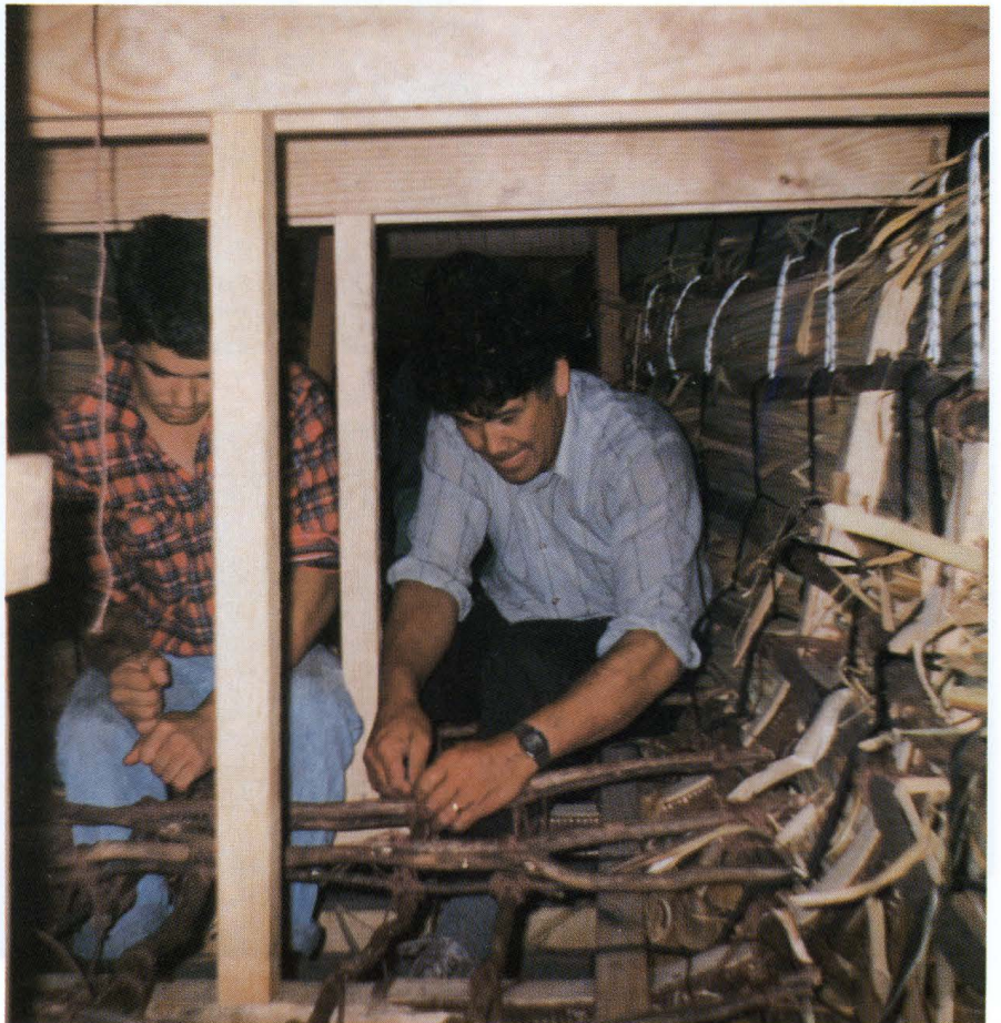
Phillip Preece and Mana Cracknell lashing floor braces.
